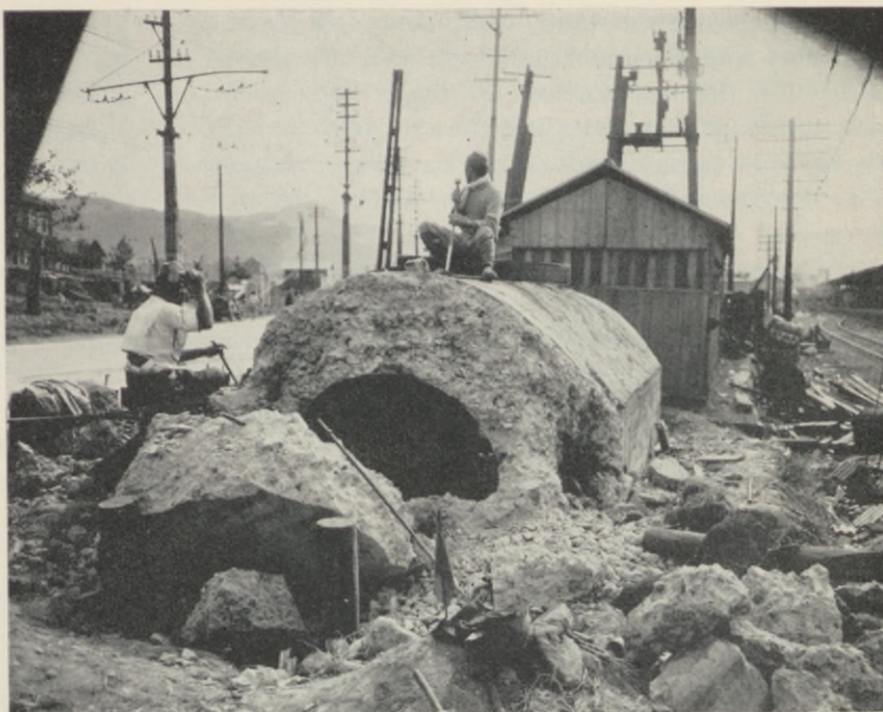
Photo 29. Workers breaking down a concrete shelter built for and by the railroad employees. Nagasaki Station, Nagasaki City.
